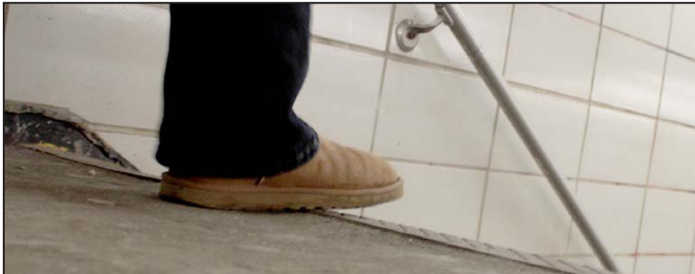
Image 8: A photo we took showing a 1/8-inch raised lip on a subway station stairway aided our client to win an award of $100,000.
