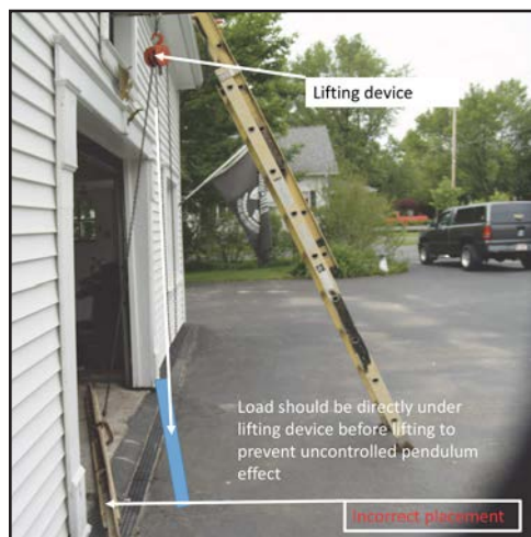
Image 1: This is a still shot from a video that was made to reconstruct the accident. It helped earn our client $11 million.
